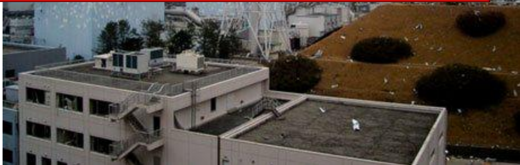
#3 Loss of cooling
