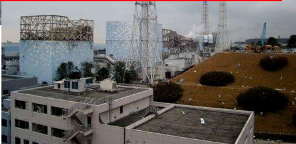
#3 Loss of cooling
