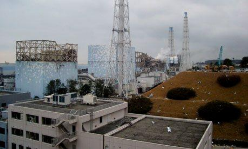
#3 Loss of cooling
