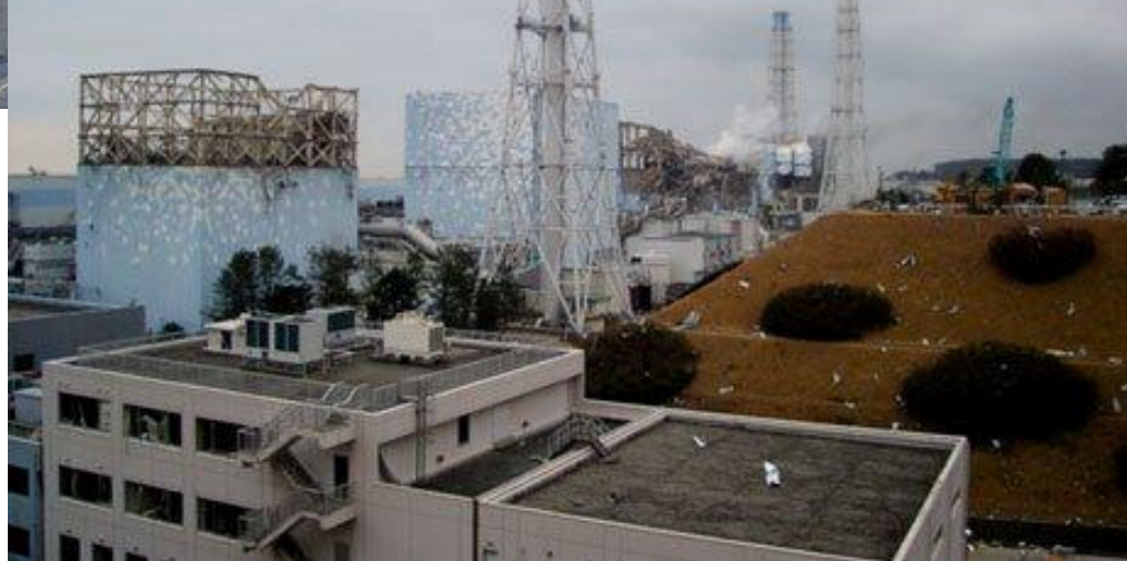
#3 Loss of cooling
